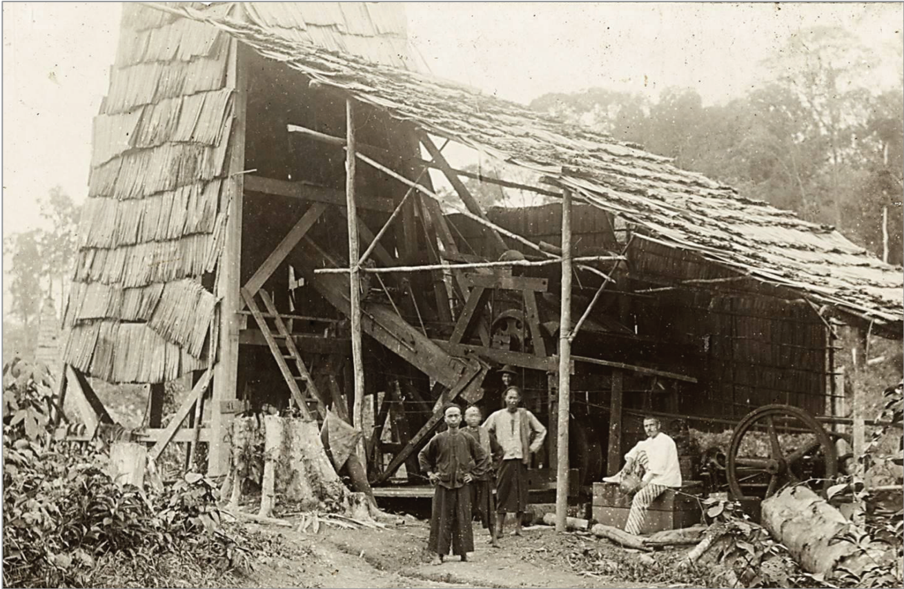
Fig. XIX.10. A Dutch drilling supervisor and three Chinese laborers at a 'Canadian-type' cable tool rig at the Babat 34 well of the Moeara Enim oil company, around 1902 (Coll. KITLV 31921, Leiden). The Babat field is listed as a 1902 discovery and became the second largest oil field of the Muara Enim Maatschappij, after Kampong Minyak. About 40 wells were drilled in the early 1900s and it produced 8-9 million barrels of oil, which was quite significant at that time. It is located west of Sekayu near the Musi River. The oil was piped to a refinery at Plaju near Palembang.
