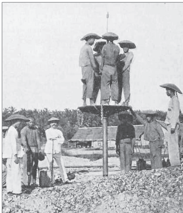
Fig. XV.7. A Chinese crew in Belitung, operating a manual coring tool known as a 'Banka drill' (Van den Broek, 1921).
