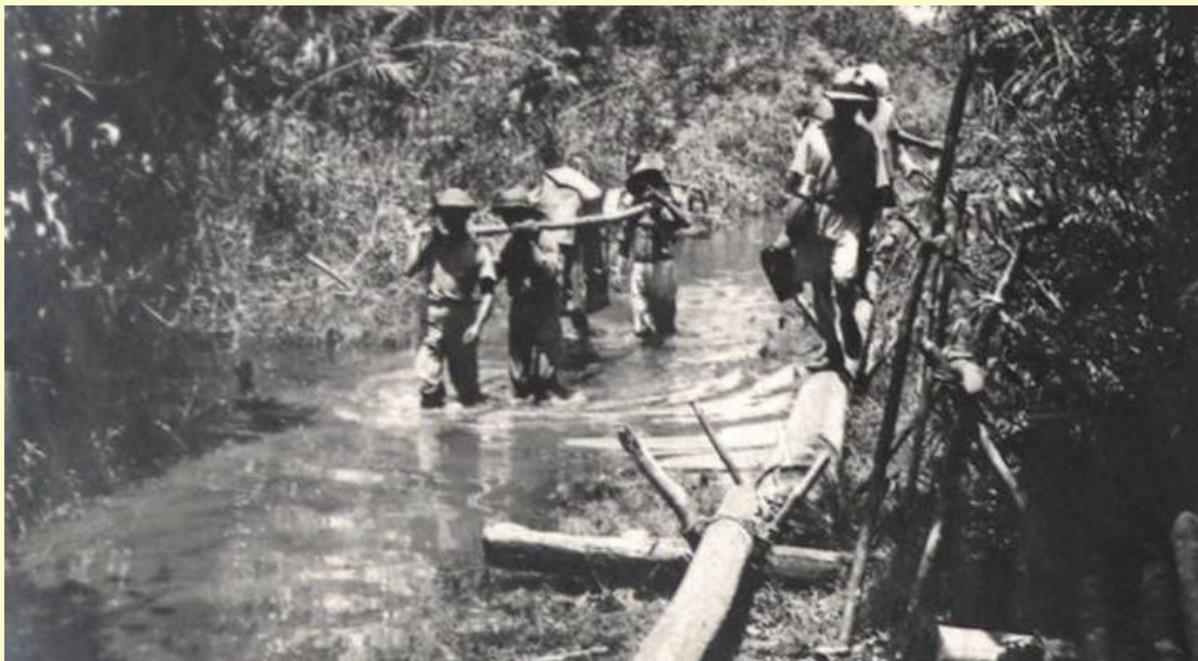
Fig. XIV.154. A gravity survey crew carrying a torsion balance along a seismic line across a swamp in Sumatra or East Borneo, 1937 (Coll. KITLV 46286). The surveys often required a crew of 100s of native workers to cut trails and move equipment through jungles and swamps.
