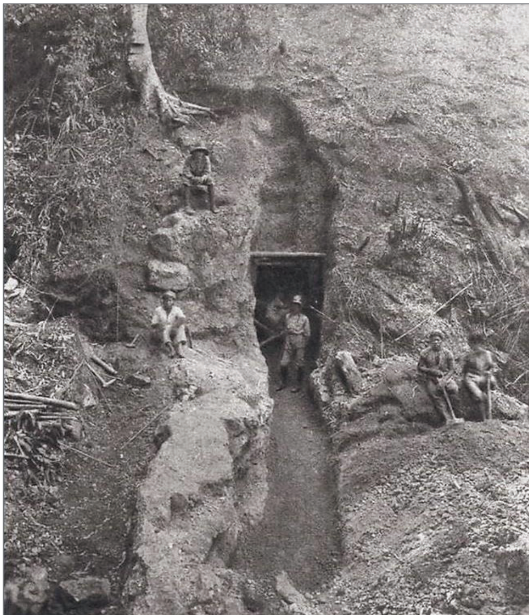
Fig. XV.112. Test excavation of a gold-silver bearing quartz vein at Tji Bodjongdeet, Jampang, West Java, during a government-directed survey in the early 1920s (Dienst van den Mijnbouw 1924, Verslagen en Mededeelingen 16). None of the mineralized veins identified and evaluated was deemed to be of commercial interest.
